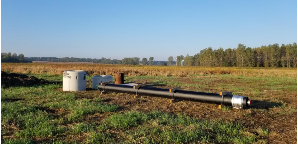
The meter pit and riser for well #11 has arrived on site.
