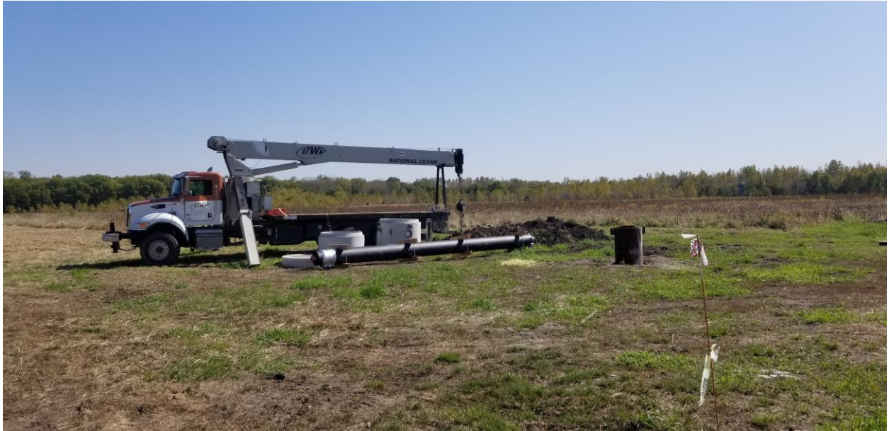
Brotke was back onsite to prep the riser for installation
