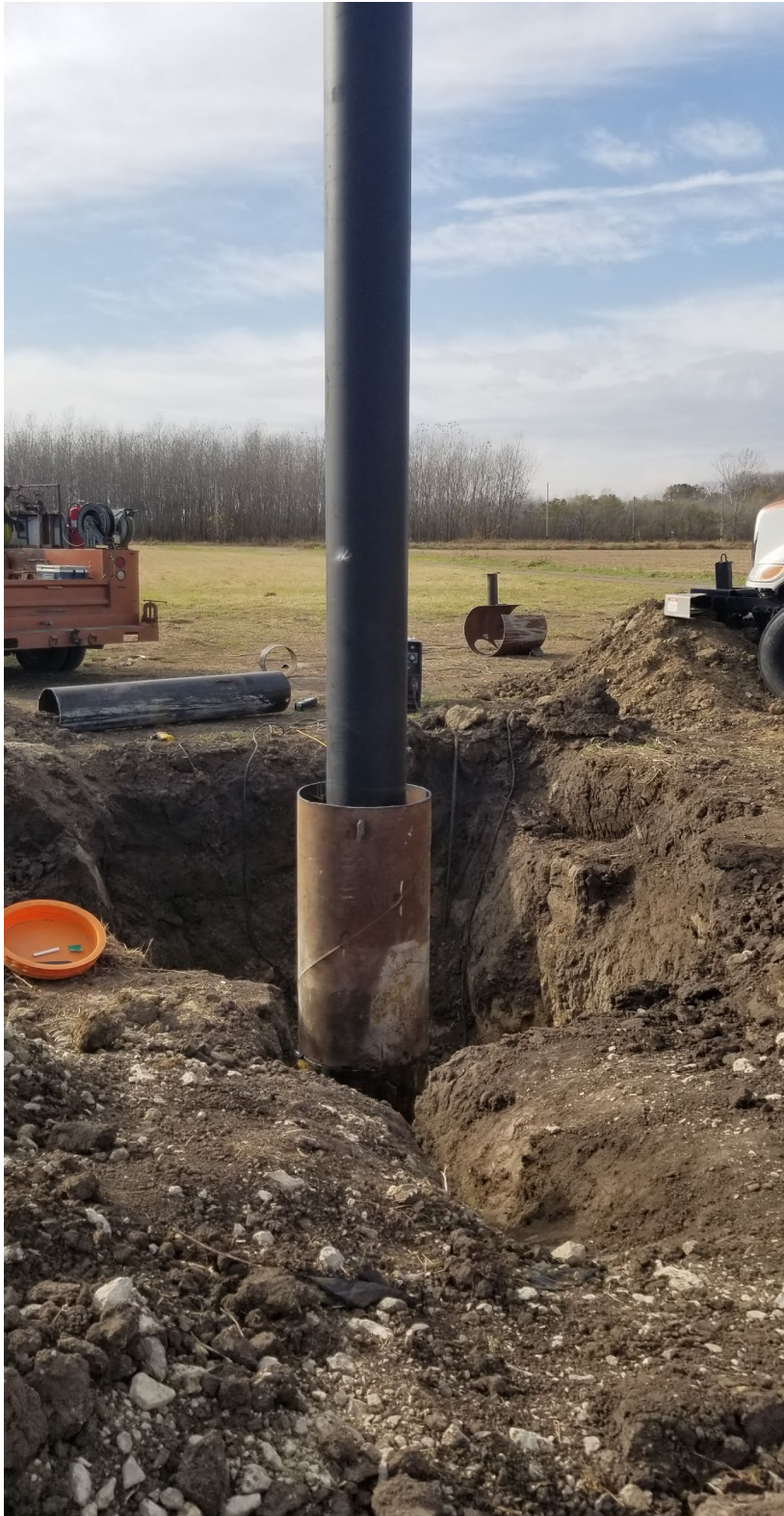
Brotke has installed the next section of casing for well #11
