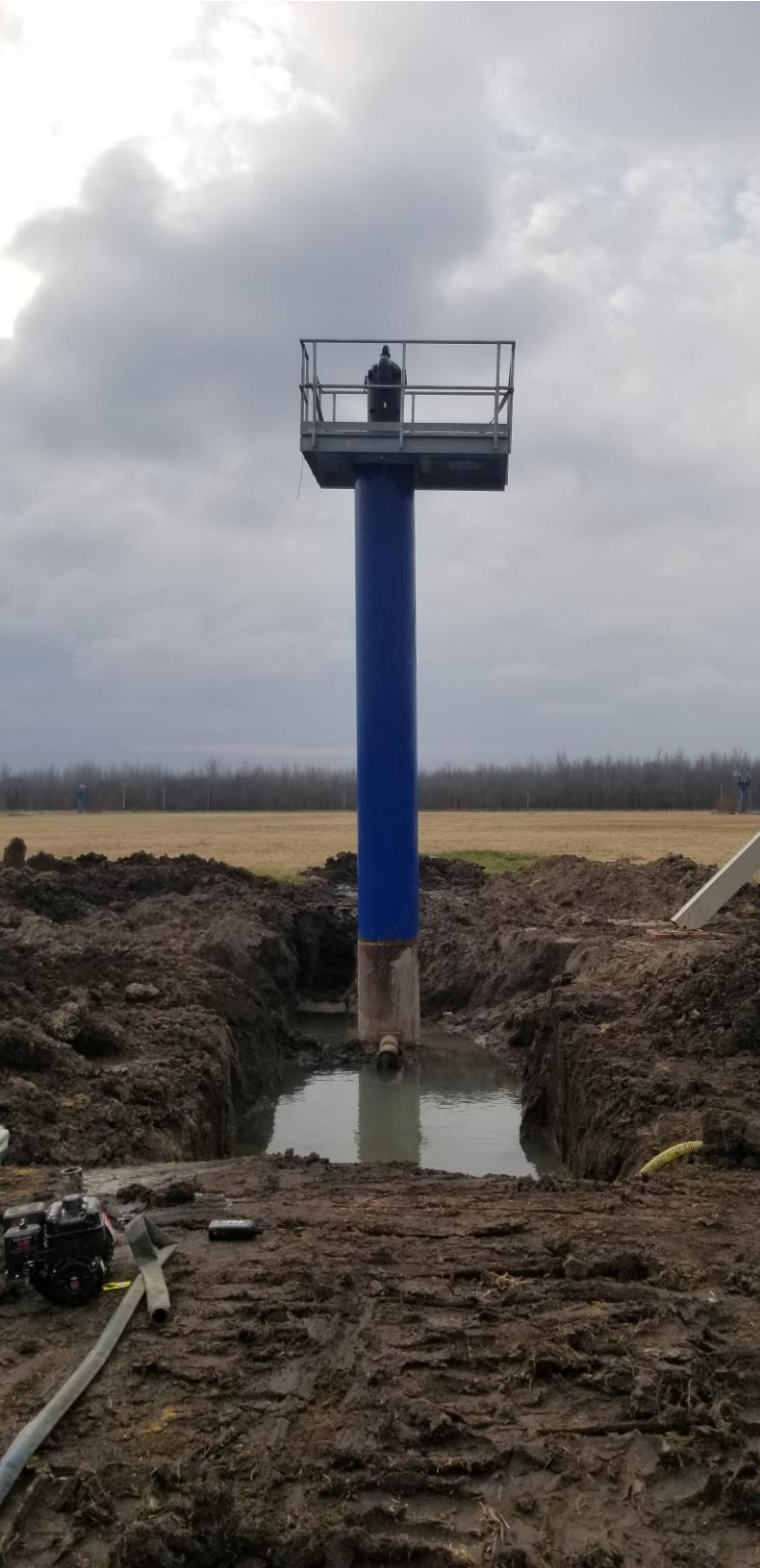
Well #11 platform has been rough installed.
