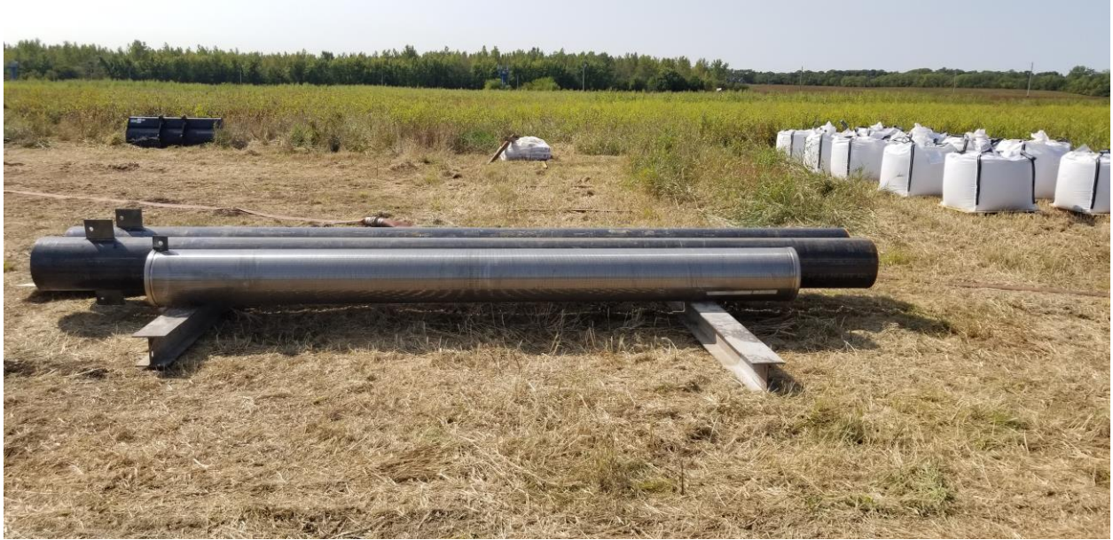
New screen and media on site
