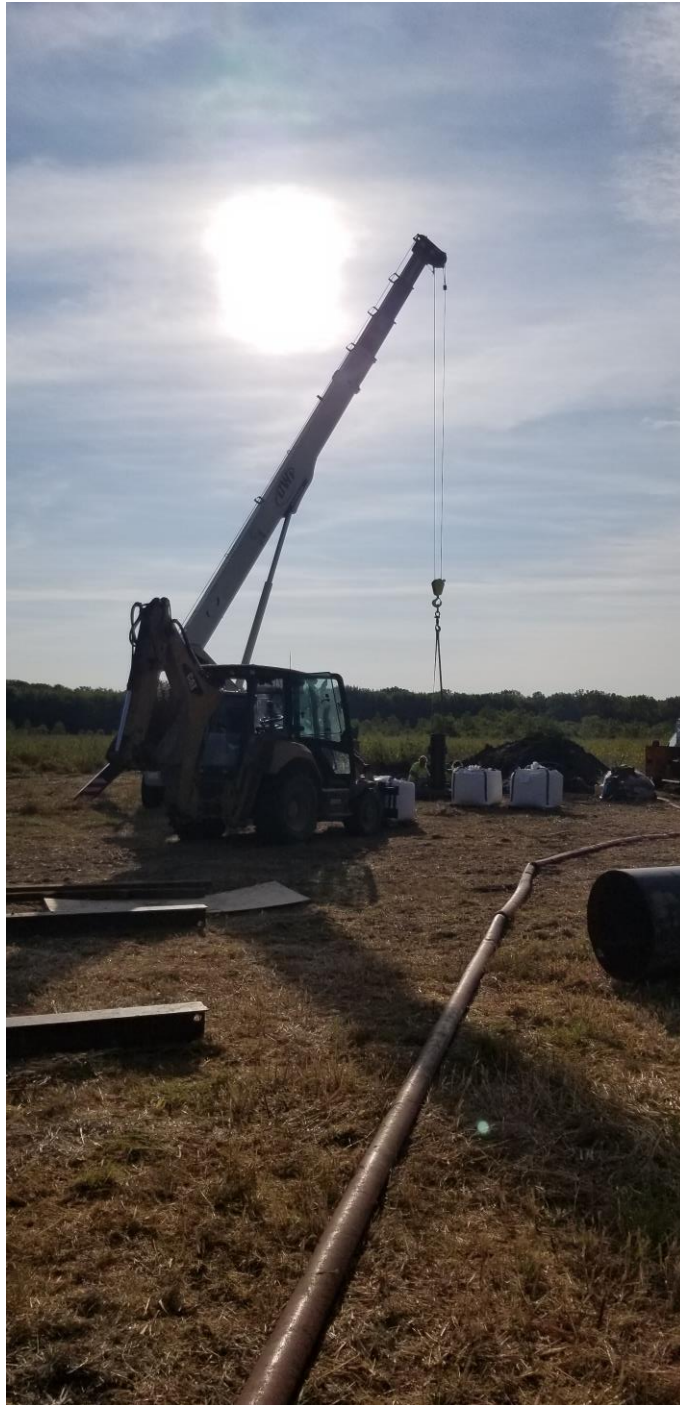
Brotke setting the screen in place for well #11
