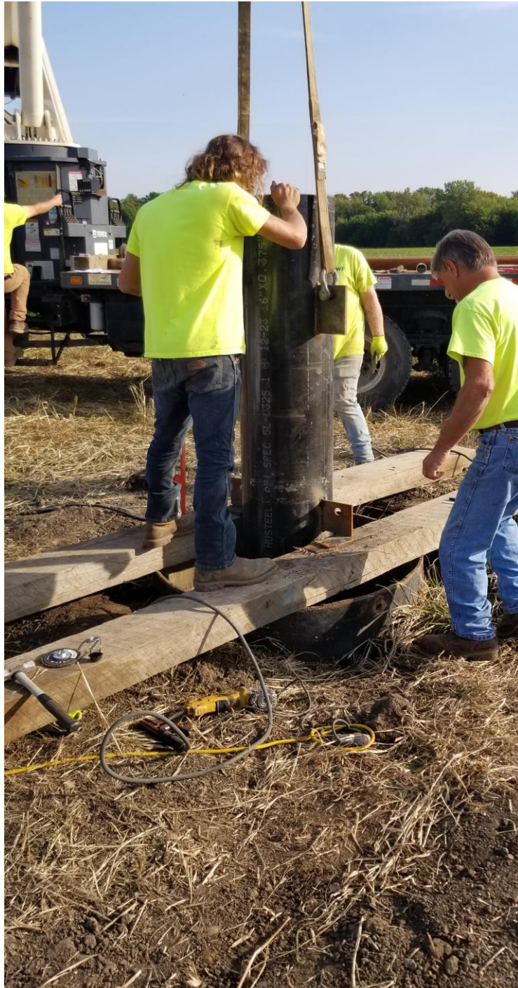
Leveling and centering the screen.
