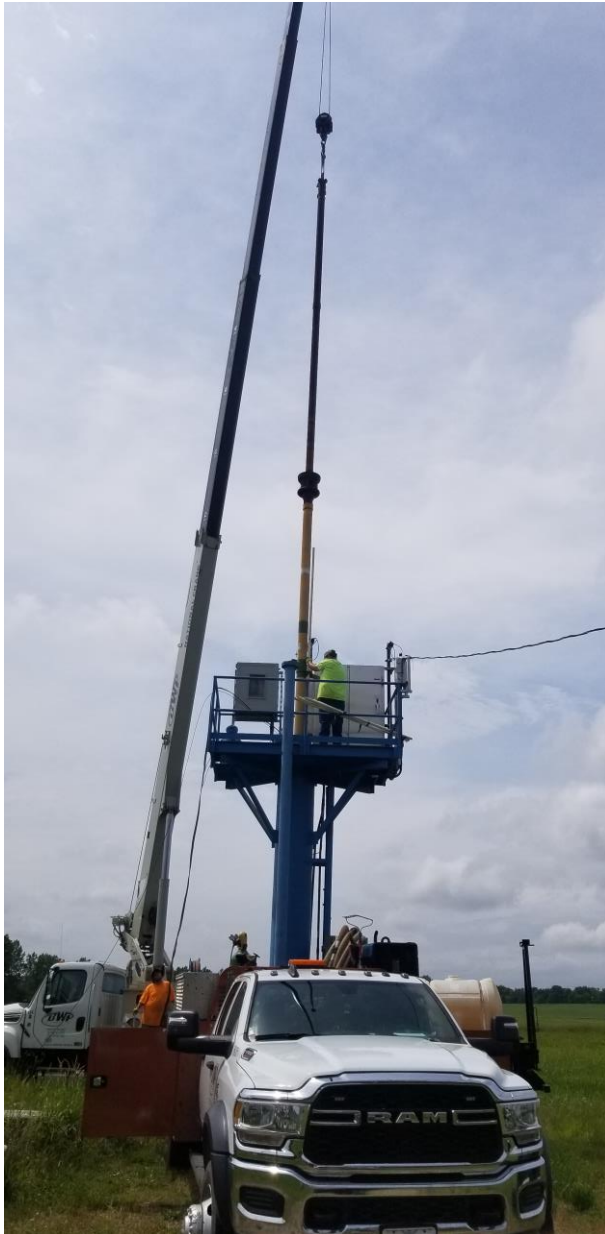
Brotke pulling well 5 to install the new transducer
