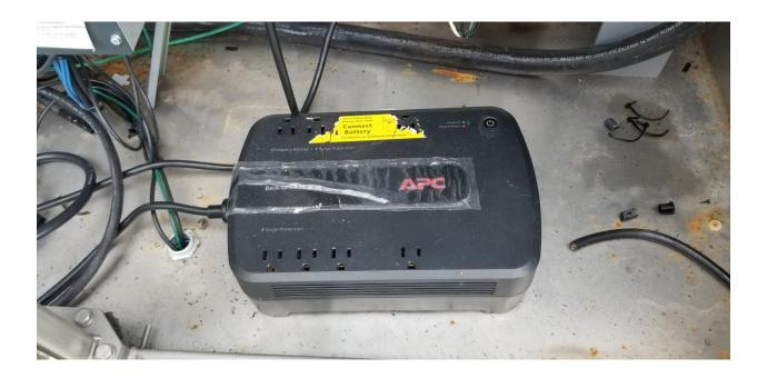
We received a comm loss alarm from well #5 in the evening. Upon inspection it was found the battery had not charged properly and had to be reset.
