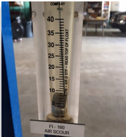
September 3, 2015 – Repair of an air regulator on Filter Bank #1 broken.
