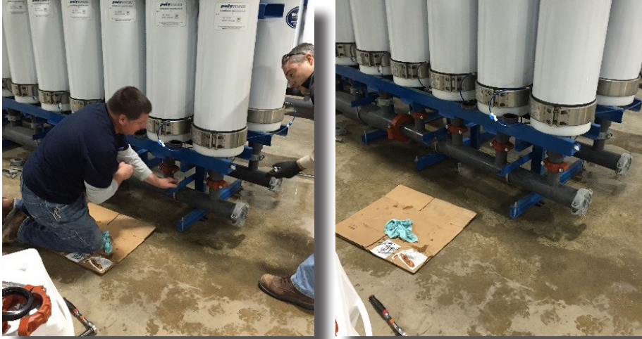
March 2016 – Repair of leak on the lower manifold on Bank#1.
